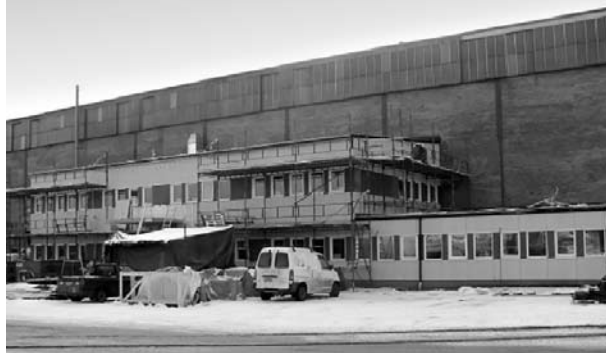
Boxholm: New office building under construction
