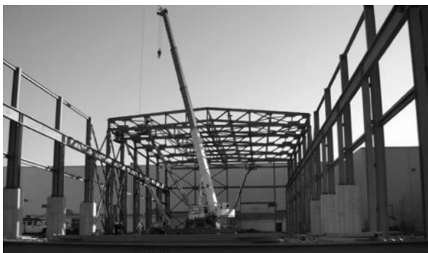
A. Finkl & Sons: Construction of the new steelworks in Chicago
