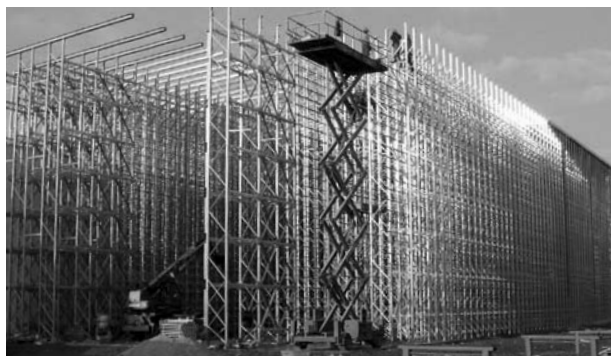
Ugitech: Modernisation of the warehouse at Grigny
