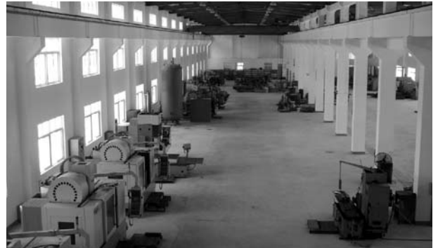
SCHMOLZ + BICKENBACH Distribution International: New warehouse at Ninghai (China)
