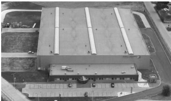
SCHMOLZ + BICKENBACH Distribution Europe: New warehouse at Myslowice (Poland)
